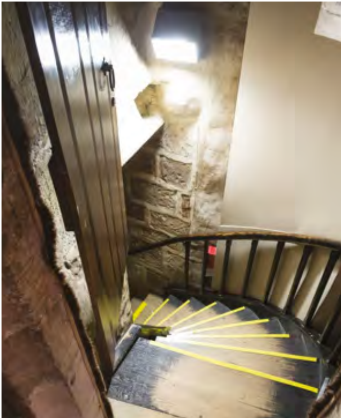
Higher lighting levels may be needed on steps and stairs.
