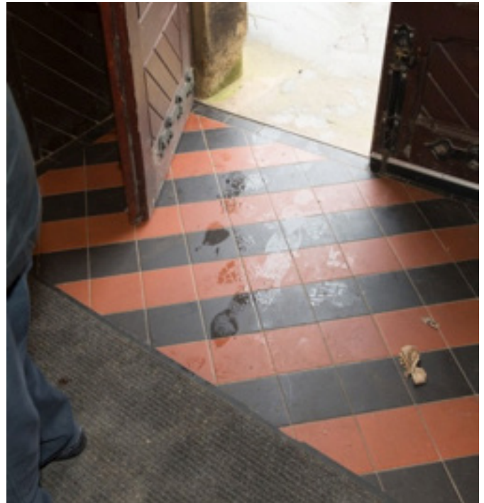
Providing and positioning absorbent entrance matting properly will reduce the risk from walk-in contaminant.
