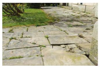
Broken paving should be noted during routine maintenance checks and suitable precautions taken until any damage can be repaired.
