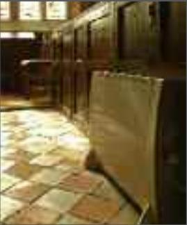
If portable heaters are required they should be of the convector or fan assisted type with a thermostatic cut out.
